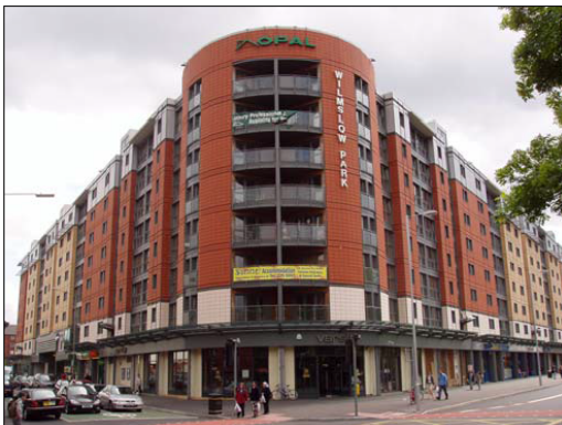
Figure 20 Typical podium structure in which seven storeys of residential units are supported on a composite frame below.
