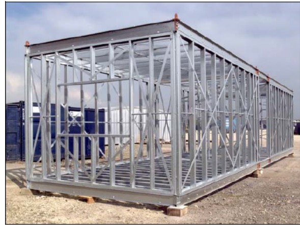
Figure 6 Long module with a corridor
