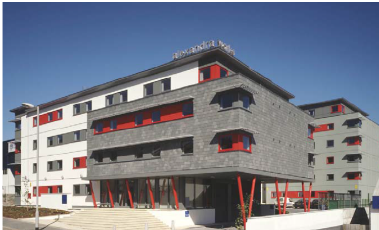
Modules supported by inclined tubular columns
