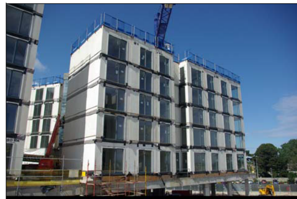
Figure 22 Modular units supported by a podium.
