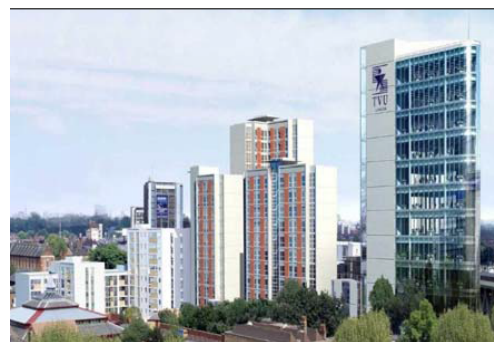
Figure 27 Concrete core can be used to stabilize 17 stories of modules
