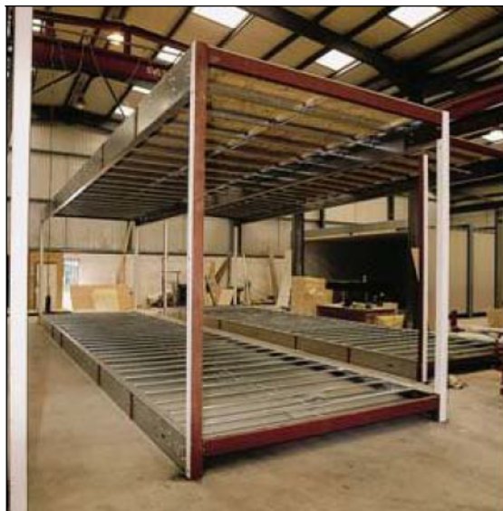
Figure 11 Primary steel frame used in an open-sided module
