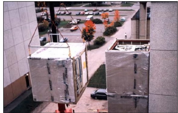
Figure 10 Open-sided bathroom modules being attached to an existing building
