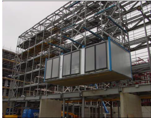
Figure 21 Installation of modules behind external steel framework.
