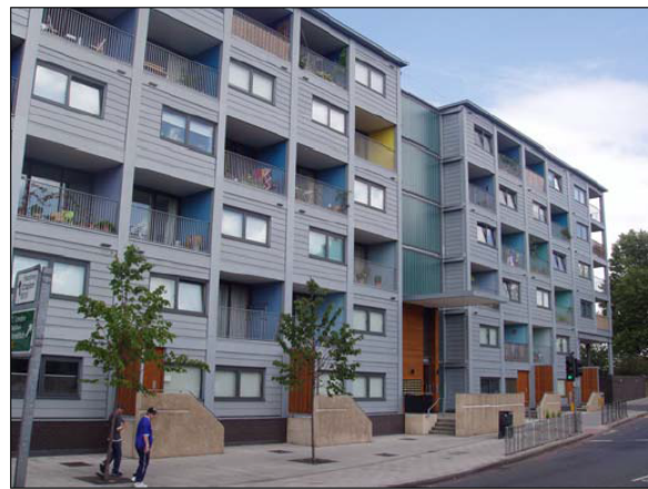
Figure 4 Image showing integral balconies
