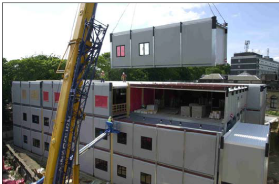
Figure 15 Modular hospital building during installation of open-sided modules
