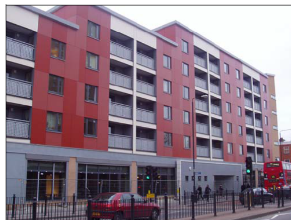
Figure 23 Mixed use of stabilising frame and modules in a residential project.
