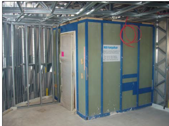
Figure 29 Toilet 'pod' used with light steel framing
