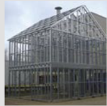
House using light steel framing for walls, floor and roof
