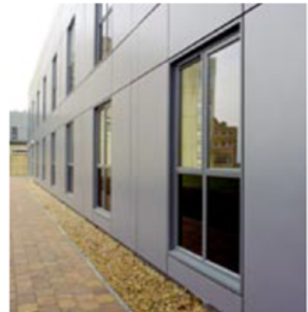
Steel cassette attached to light steel frame
