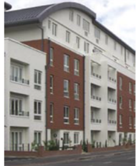
Insulated render attached to light steel frame
