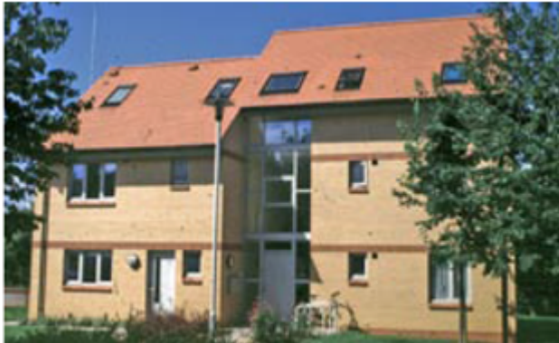
Finished building used for long term monitoring
