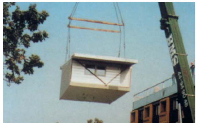
Modular roof-top units being lifted into place
