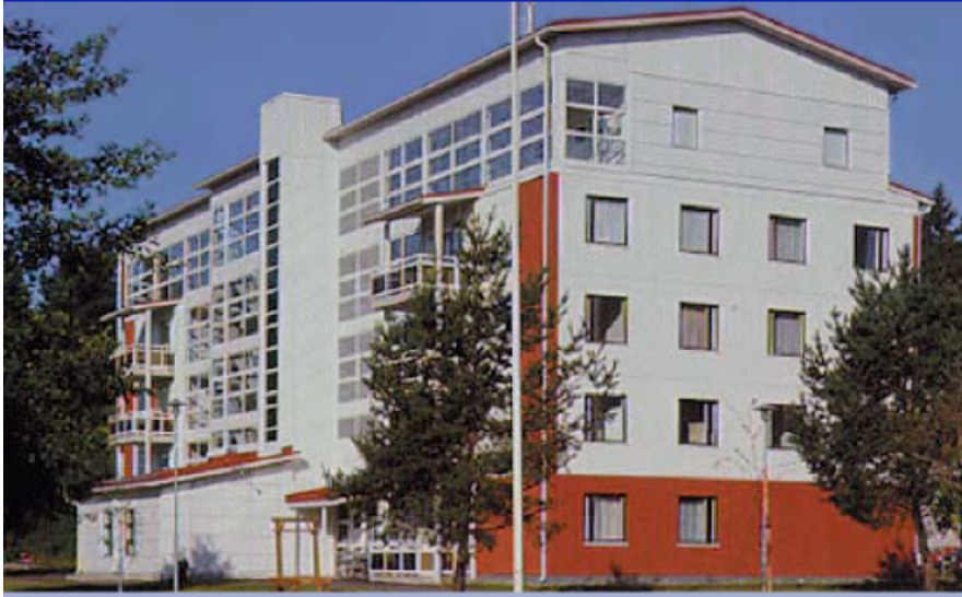
Roof-top apartments using modular units
