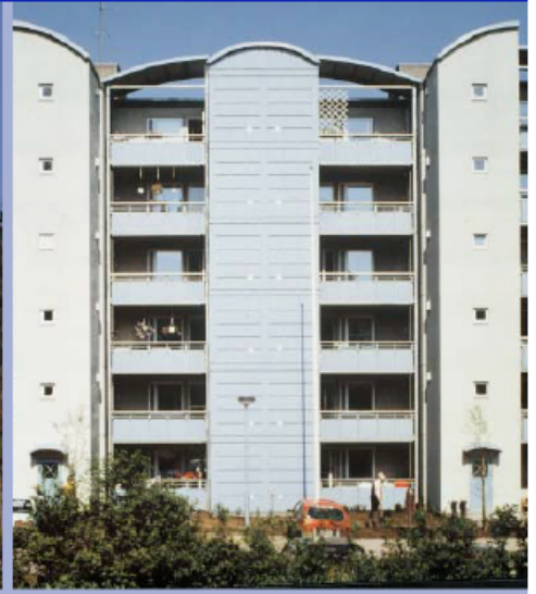
Pre-fabricated balconies and modular units
