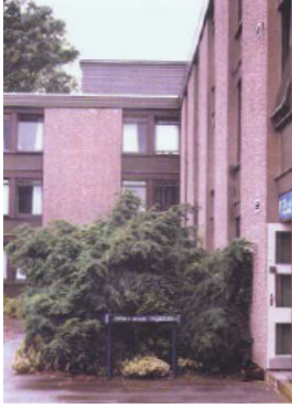
Original view of building.
