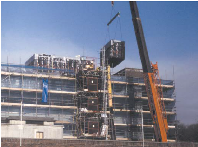
Roof top modules being lifted into place.
