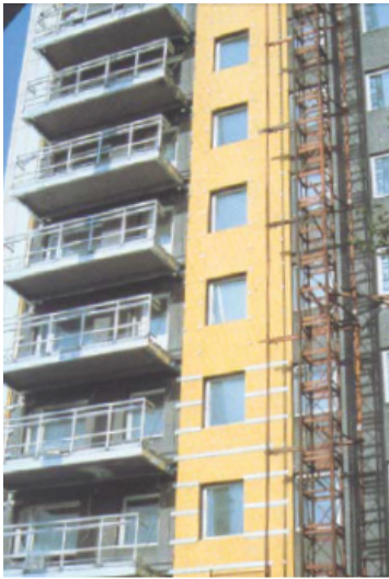
New balconies and over-cladding, Finland.
